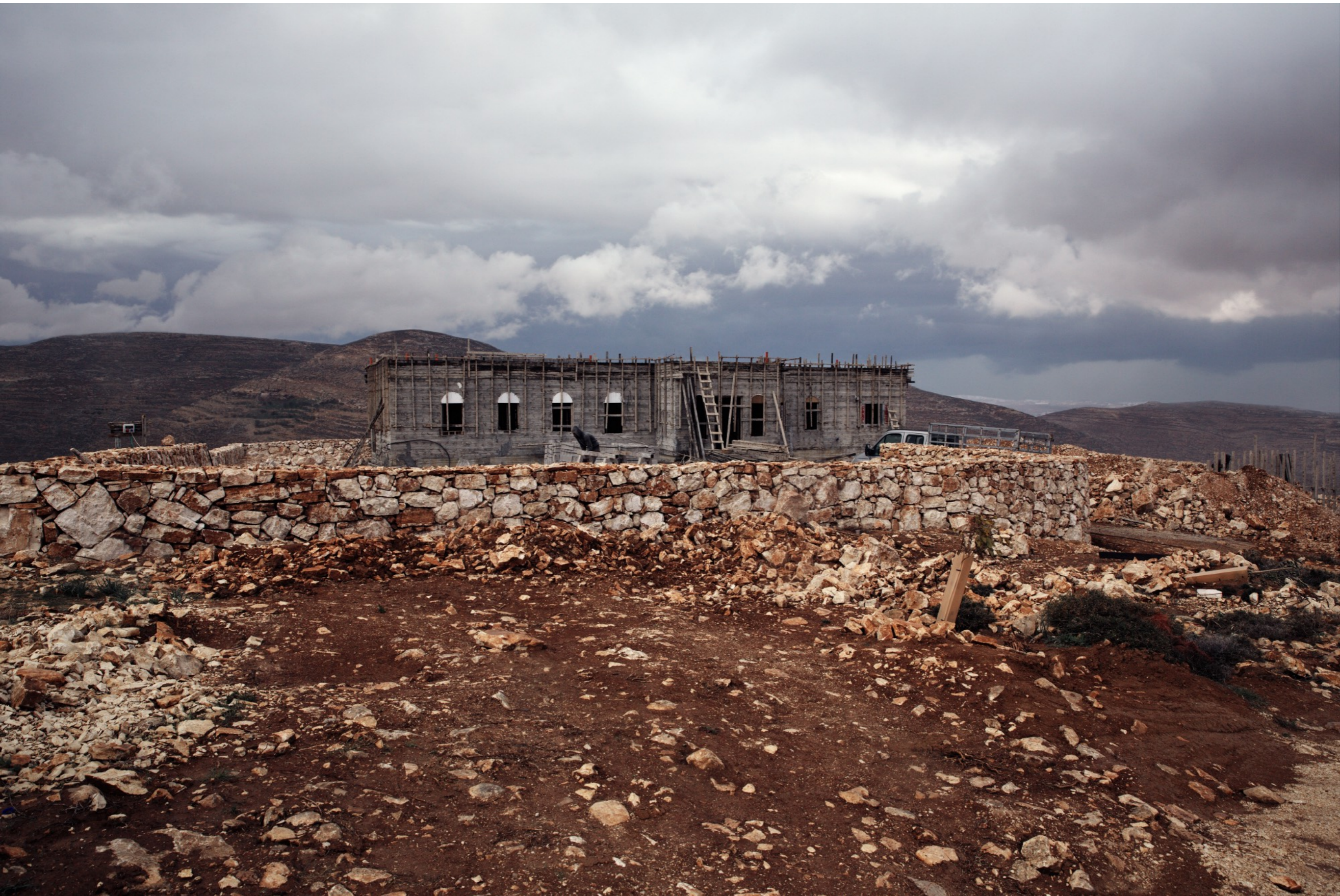
His friend's home under construction.
