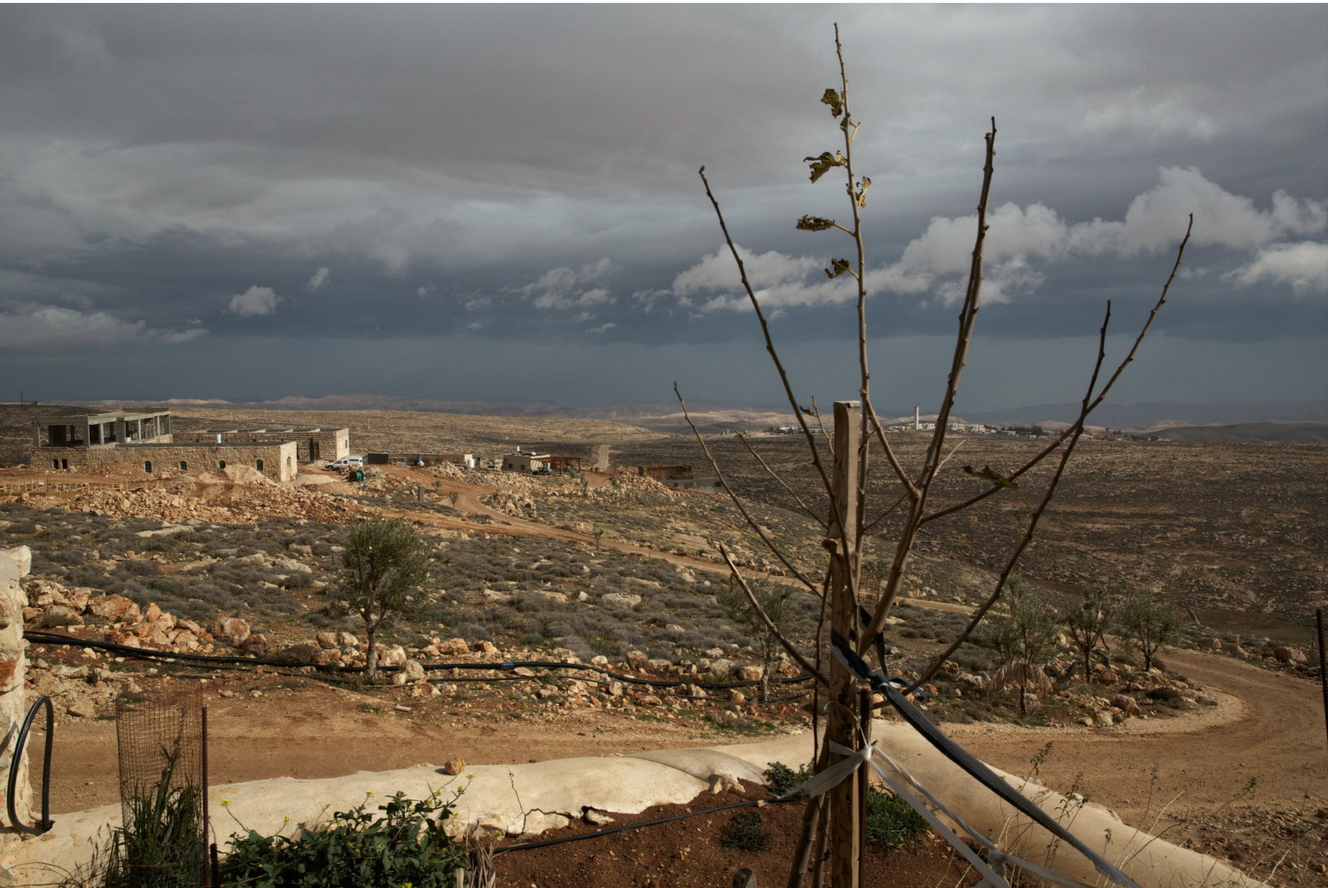
Boutique hotel under construction.
